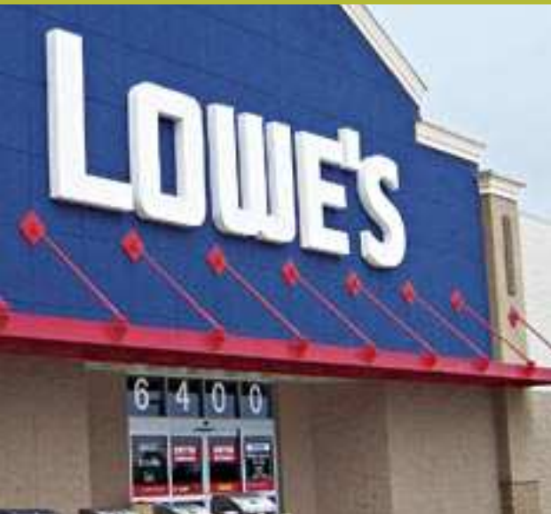
Lowe's LEEDS (Leadership in Energy & Environmental Design) Gold Award Store – Austin, TX
